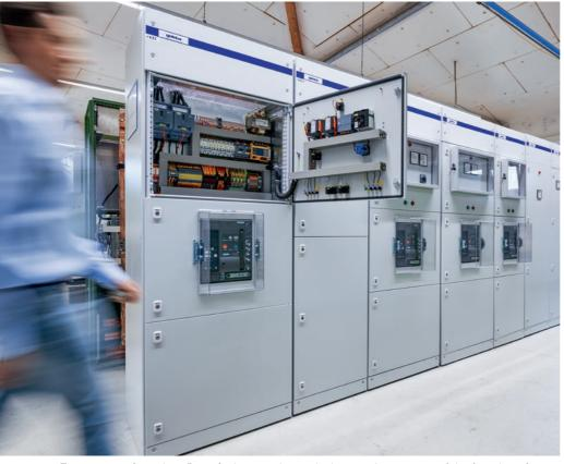
**Form separation,** class B arc fault protection and other requirements – gefeba faced a raft of challenges in the switchgear project for thyssenkrupp Steel Europe.
